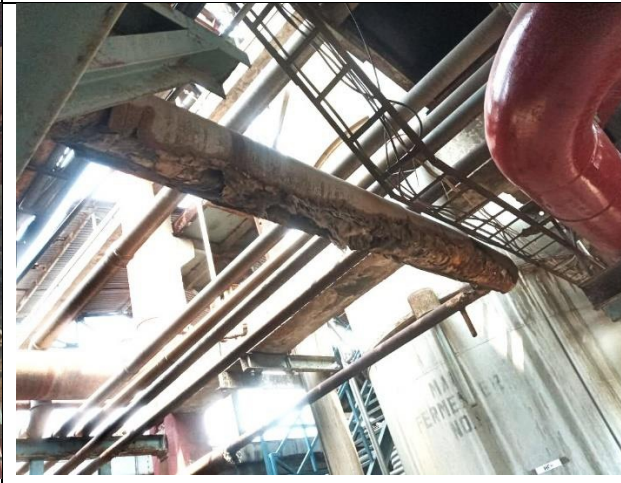
Rusted pipes of the plant exposing asbestos hazard
