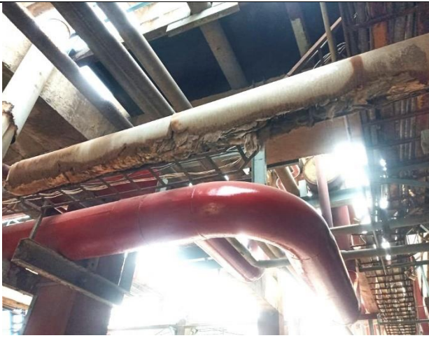
Rusted pipes of the plant exposing asbestos hazard
